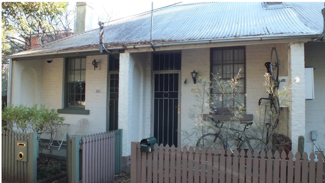
Figure 21 — South elevation of attached cottages – from left to right - Nos 89E and 89D. The timber framed double-hung sash windows on both cottages are 6-panes per sash. The doors have fanlights over. The verandah floor finish is painted concrete (Source: NBRSPARTNERS, May 2015)
