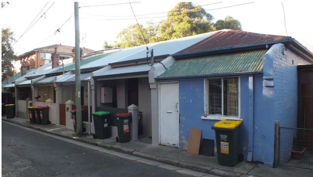
Figure 29 — View looking east along James Street to the north elevation of (from left to right) Nos 11, 13, 15, 17 and 19 James Street showing masonry painted and rendered, hipped roof in corrugated metal and chimneys missing from cottage Nos 15, 17 and 19 James Street. No 19 James Street has an infilled verandah and the metal roof is corroded. The west elevation of No 19 James Street is painted face brick (Source: NBRS+PARTNERS, May 2015)
