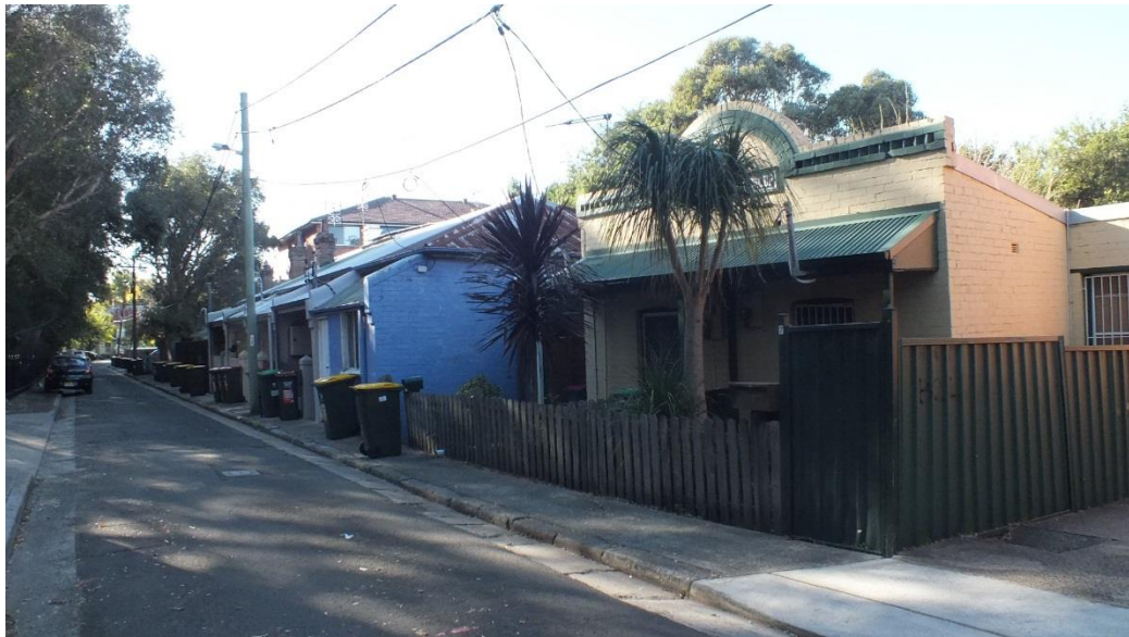
Figure 30 — View looking east along James Street showing the street context of an Inter-War painted face-brick building housing the 1 st Sydney Scout Group, adjoining the group on the east. A three-storey, mid-20 th century face-brick flat building is evident in the distance and to the east of the subject row of single-storey terraces (Source: NBRSPARTNERS, May 2015)
