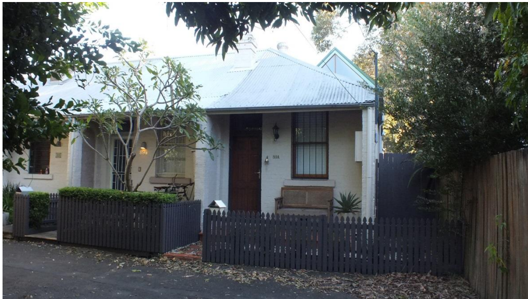
Figure 23 — South elevation of attached Victorian style cottages – from left to right - Nos 89C, 89B and 89A. The timber framed double-hung sash windows at No 89A are 1-pane per sash. The verandah floor and paving to No 89A are finished with later addition terracotta tiles and glazed gable additions are evident at the rear of the cottage (Source: NBRS+PARTNERS, May 2015)
